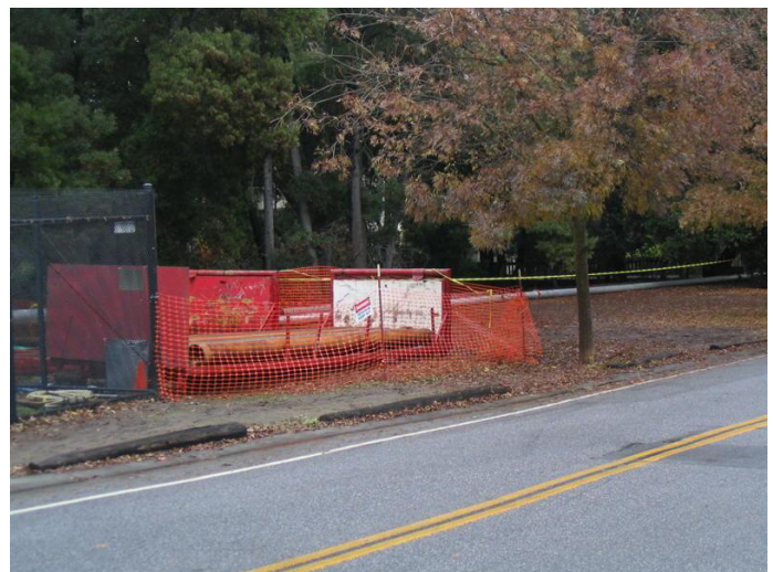
Illustration F: Example of Equipment Staging at the Well Site, 2010
