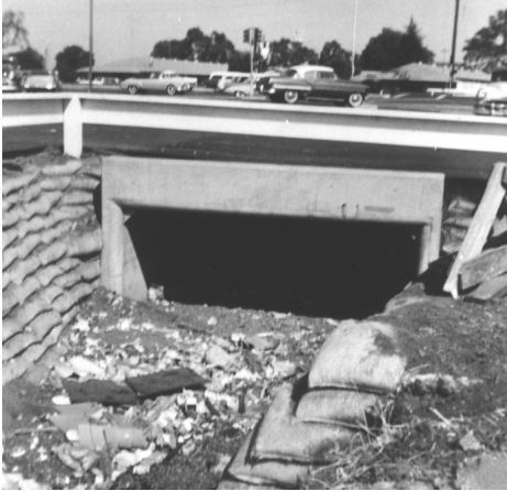
Previous entrance to the culvert under El Camino Real when Barron Creek was still an open ditch along Los Robles Avenue. Fall 1958.
