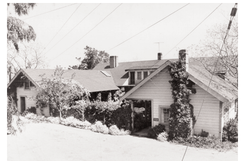
This shows the west side in 1963—there have been no major changes since, except for vegetation growing up.
