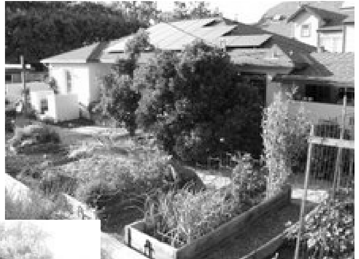
The home of Romie and Mark Georgia features a sustainable garden as well as photovoltaic panels
